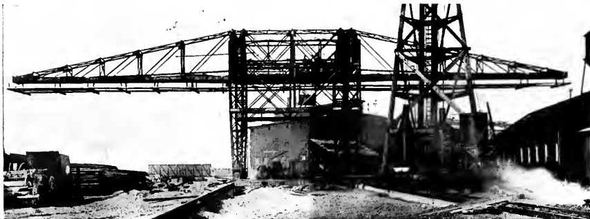
The large gantry installed to handle material in the plate and shape storage space of the new Alameda branch of the Union Iron Works Company.
